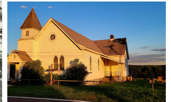
Church of the Brethren in Farmington, Pa, built in 1919, is the church where Weller's father ministered.
